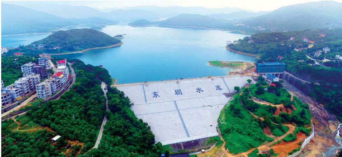
Comprehensive water environment treatment for Dongzhen Reservoir
